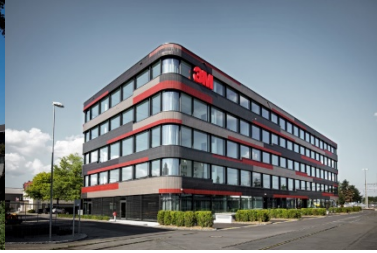
3M EMEA headquarter in Langenthal, Switzerland. (Photo: 3M)
